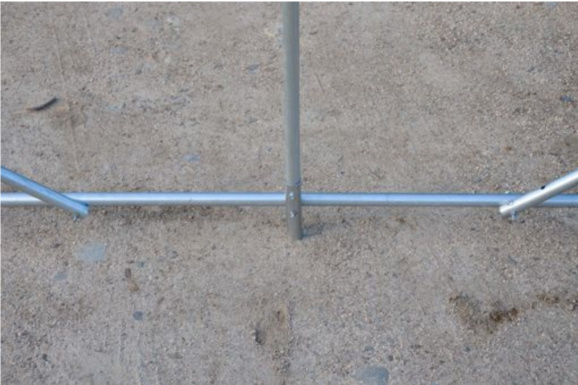
Base connector with diagonal braces.
